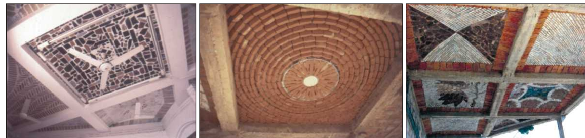
Photographs courtesy: Anangpur Building Centre
