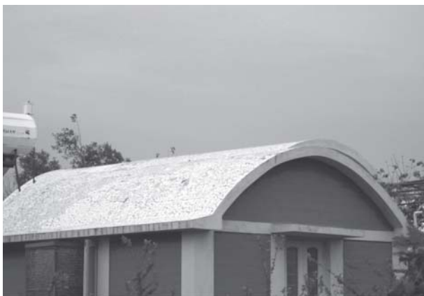
Fig. 1– Guna tile vaults at GSV campus, Wardha
