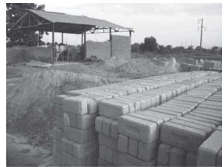
Khaparkheda fly ash brick unit
